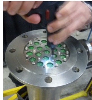
Installation and screwing of the tightening plate
