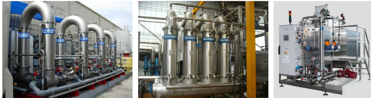
Pictures of our installation with Pleiade® and MP4® membranes
